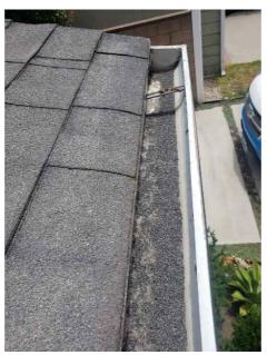
**Coverings: Material** Wood, Shingle All this pictures needs action Metal flashings not seal to tile roof
